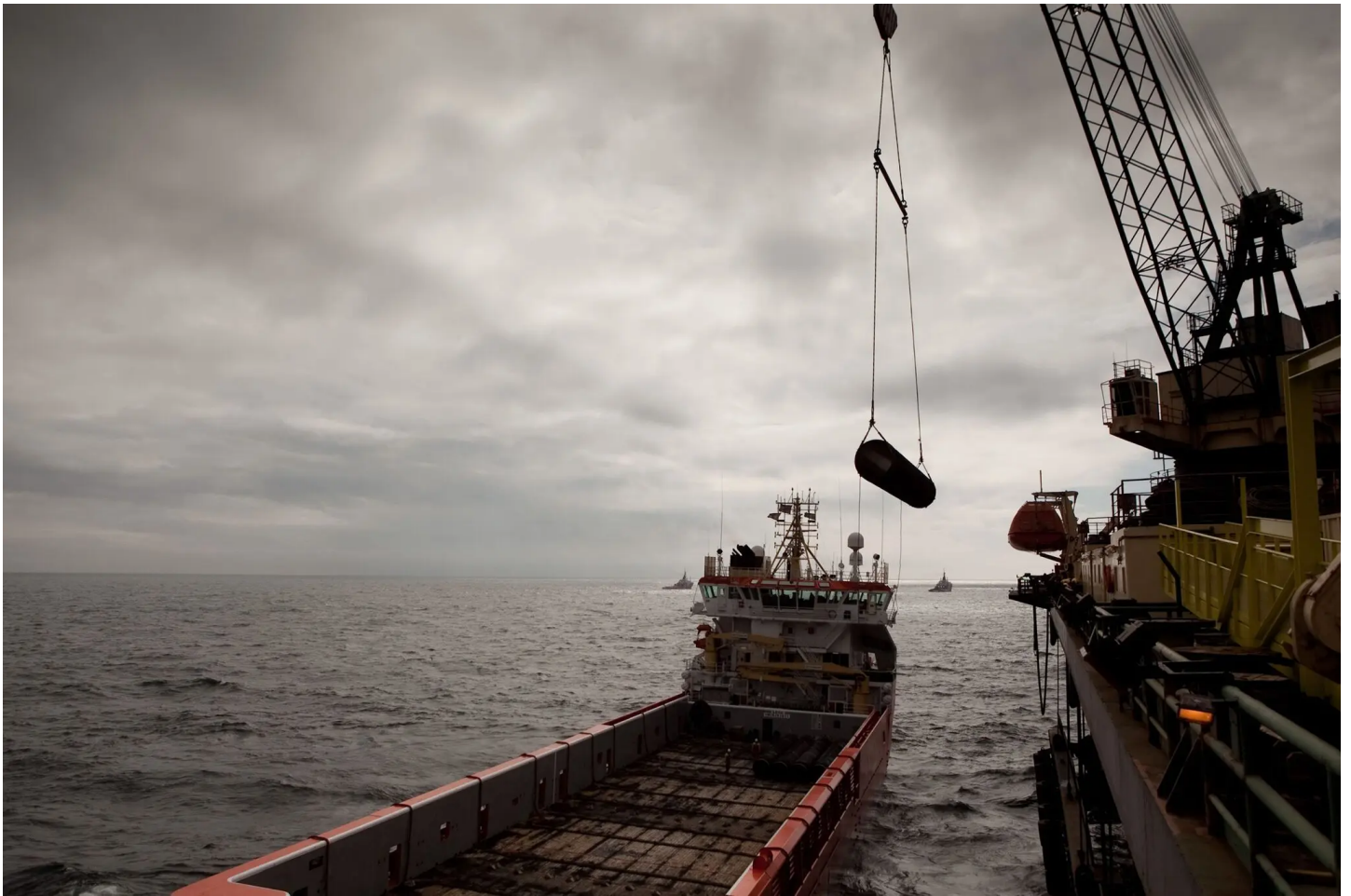
A section of the Nord Stream 1 gas pipeline during construction in the Baltic Sea in 2011. Timothy Fadek/Bloomberg
